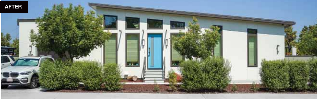
The Huang residence: an innovative take on Joseph Eichler by the BONE Structure design team
