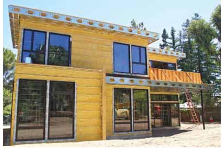
Left: The framing system for Bone Structure homes is made of steel tubes manufactured in factories and designed to connect together on-site. Courtesy Bone Structure. Right: Bone Structure built its first California home, shown here during construction, in Stanford in 2016. The home's frame was built using laser-cut steel and spray foam insulation. Photo by Veronica Weber. Bottom: Local residents had an opportunity to tour this home under construction in Palo Alto in late 2022 during an open house highlighting the company's framing system. Courtesy Bone Structure.
