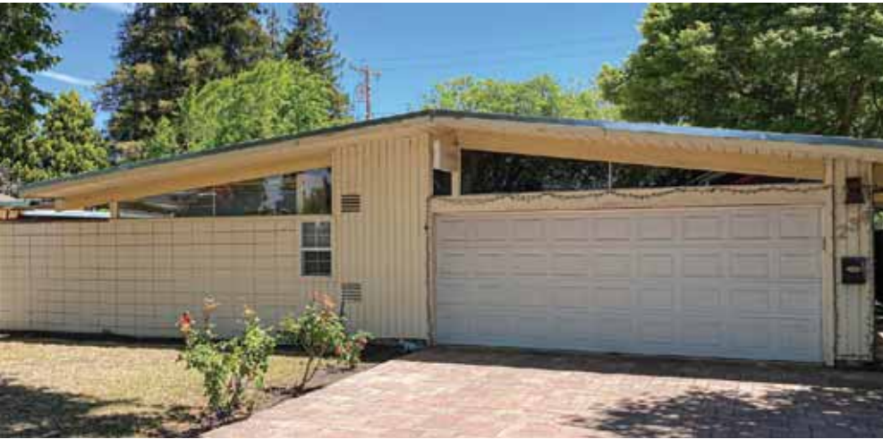
Homes in Joseph Eichler's Greenmeadow subdivision were offered in six floorplans. They all shared similar exterior features, such as clerestory windows, as show in both photos above. Courtesy Bo Crane. Facing page, bottom: The community center, built as part of the planned subdivision in the 1950s, remains the center of neighborhood activities. Courtesy Bo Crane. Facing page, top: Even remodeled homes in the neighborhood, like this one, have retained much of their original features. Photo by Veronica Weber.
