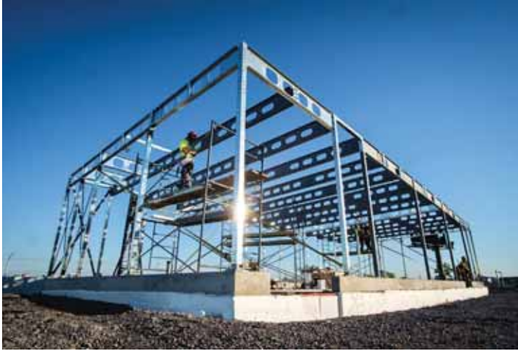
Left: The framing system for Bone Structure homes is made of steel tubes manufactured in factories and designed to connect together on-site. Courtesy Bone Structure. Right: Bone Structure built its first California home, shown here during construction, in Stanford in 2016. The home's frame was built using laser-cut steel and spray foam insulation. Photo by Veronica Weber. Bottom: Local residents had an opportunity to tour this home under construction in Palo Alto in late 2022 during an open house highlighting the company's framing system. Courtesy Bone Structure.
